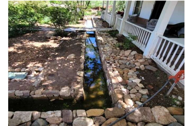
The historic acequia, reconstructed in 2023, was created to irrigate the flower garden in the 19th century. Water saving drip irrigation is used today.
