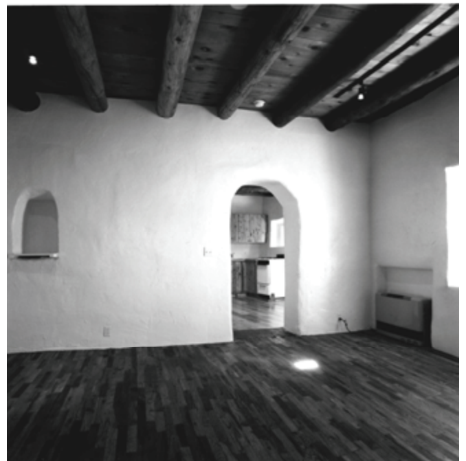
The Garcia House, north room, after the restoration. Before the restoration, the vigas were concealed behind a drop ceiling. Photo by Hope Curtis.
