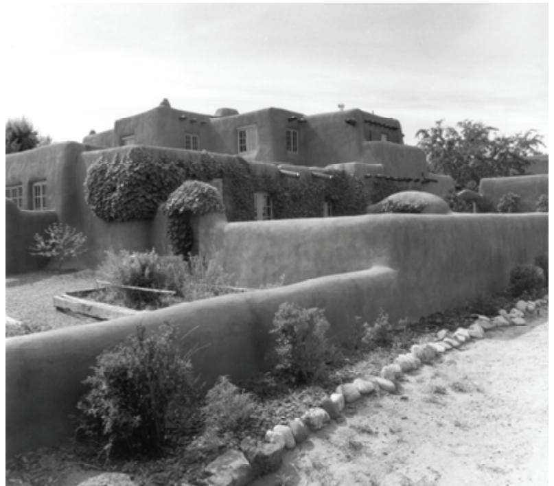
Carlos Vierra House (1918) showing portal and second-story set-back, a design element encouraged by Vierra. Photo by Vincent Foster.
