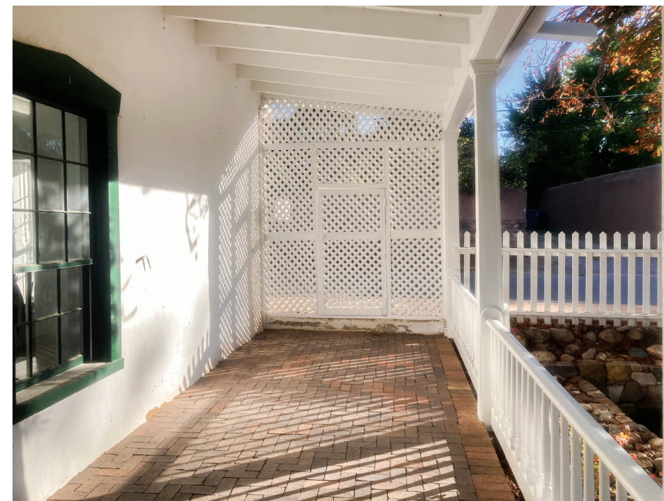
Photos clockwise: Edwin Brooks House door, renovated sala, & repainted portal by HSFF Staff.
