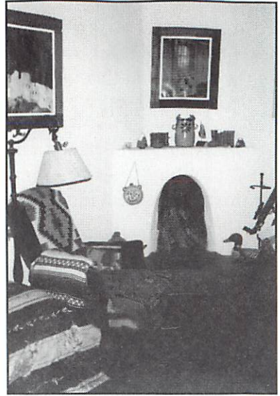
Bedroom fireplace after renovation. Photographer: Lynne Andrews.
