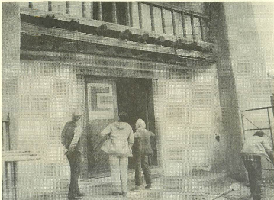
Dr. Jenkins and others inspect front of church.
