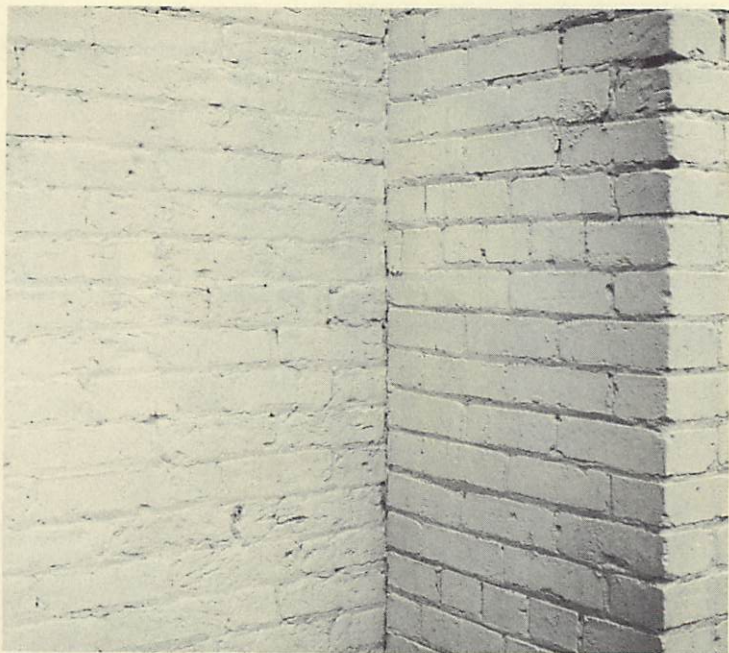
1882 Hand-moulded brick on the left used in the construction of the Hayt-Wientge Mansion and machine pressed brick on the right utilized in an 1899 addition.
