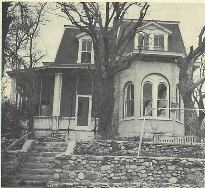
Hayt-Wientge Mansion, 620 Paseo de La Cuma Cultural Properties Review Committee and State Planning Office Photo Files, State Records Center and Archives, Santa Fe, New Mexico.
